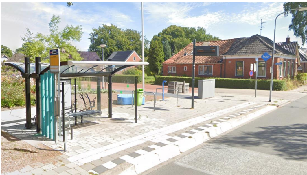
Figure 3.14: View of Siddeburen Bus Hub 98
