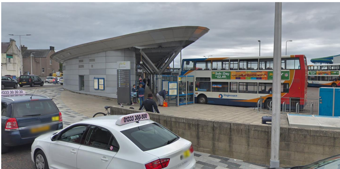
Figure 3.24: Leven Bus Interchange from Branch Street 133
